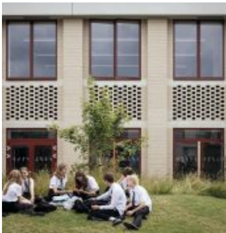
Above: The facade of the Katherine Johnson Building employs 'hit-and-miss' brickwork, as well as expressed masonry lintels and cills.
