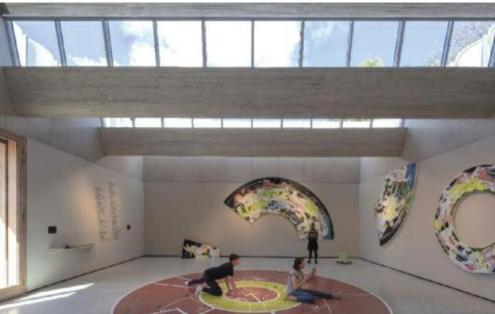
The boardmarked north-light gallery roof was cast against narrow timber battens, and is wrapped in translucent GRP.
